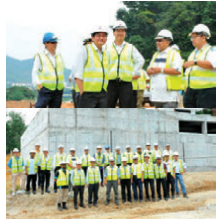
27 OCTOBER Package 1B, Langat 2 water supply scheme Site Visit by CEO of Pengurusan Aset Air Bhd
